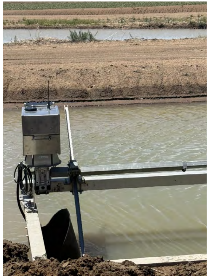
Figure 2: A rack and pinion system is used on large outlets after finding winch systems were unreliable and control devices too high above the ground – at risk of being hit by sprayers.
