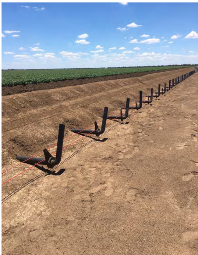
Figure 2: Smart Siphons are fitted with rotating elbows and up to 150 are connected to a common cable that is coupled to a hand winch that can be automated. Photo credit: Lou Gall.
