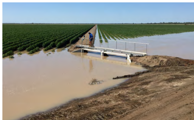
Figure 5: GL Bays releasing tailwater.
