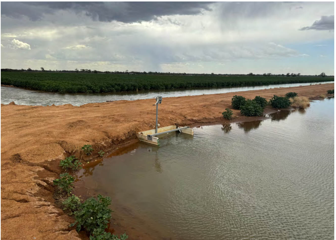
Figure 7: In a Rollover Basin, the furrow direction follows the slope of the landscape and machinery can 'rollover' the bankless channel into the next basin of the same field. In this image the road is between two basins of the same field, with a bankless channel on both sides of the road. The bankless side channel connects the basins via a pipe under the road.
