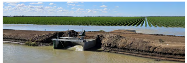
Figure 1: Pipe through the Bank is an example of a siphonless layout that has evolved as cotton growers adapt layouts to improve productivity and resource efficiency.
