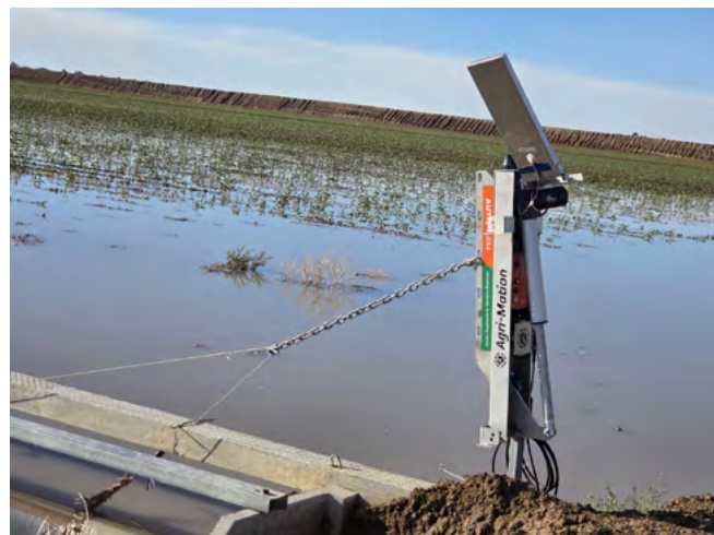
Figure 4: Linear actuator-based control solution designed to open and close inlet/outlets. Commonly these are used for smaller structures. In this case; Bluetooth and telemetry are used for communication, whilst other solutions on the market have buttons and screen to access basic-timer functionality without telemetry.
