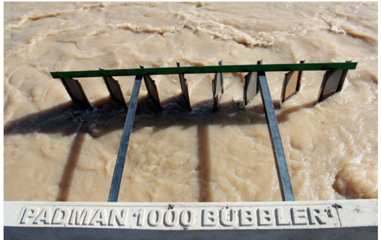
Figure 1: Padman Bay Outlet fitted with dispersion vanes.
